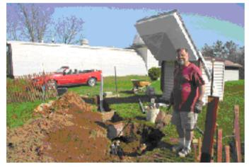
The concrete was poured in two stages. A footing for the pier is separated from the rest of the slab to reduce any vibration. The pier was welded up from scrap steel and the wedge is a spare that I had machined when I built my home observatory.
