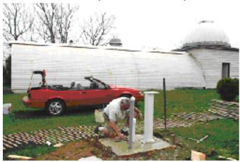
The building is a flip top design that has worked well for me for several years. The entire thing was built in my garage, complete with siding and the hinged lid. Henry and I hauled it to the observatory and anchored it to the slab. Meanwhile, Vern Hoag built a door for the new observatory and had it primed and ready for installation.
